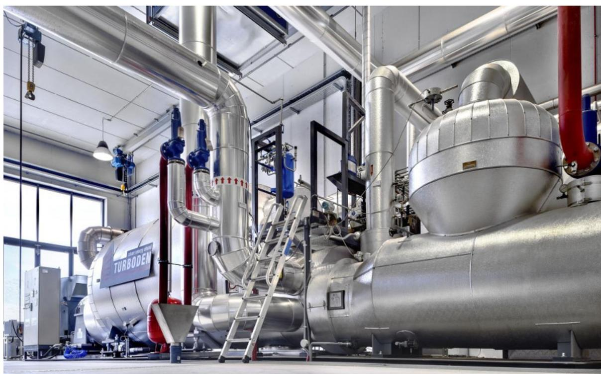
**Figure 7: 5.5MW<sub>e</sub> biomass fired Turboden ORC in Turkey**
